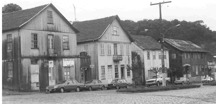
Fig. 3: Architectural and urban ensemble of Antônio Prado, landmarked in 1990. Source: IPHAN-RS archives, 1984.
