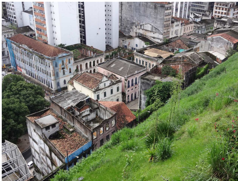
Fig. 3: The degradation of some old houses in the historical centre of Salvador (BA). Source: Author, 2013.
