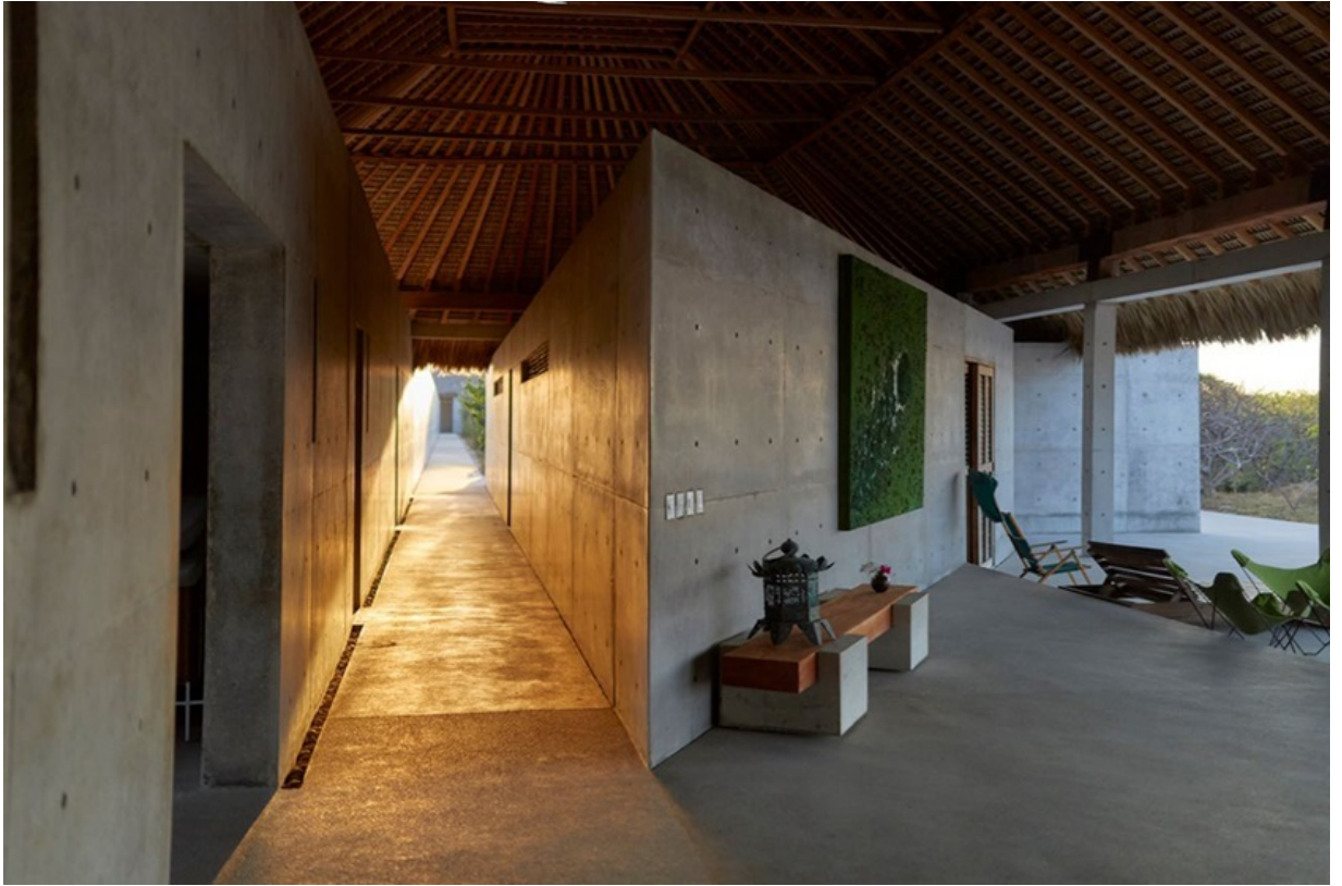
Fig. 4: View of the main building's interior. The roof is detached from the concrete beams and pillars. Source: Sergio López, 2019. Available at: https://www.sergiolopez.mx/houses/casa-wabi . Accessed 02 May 2021.
