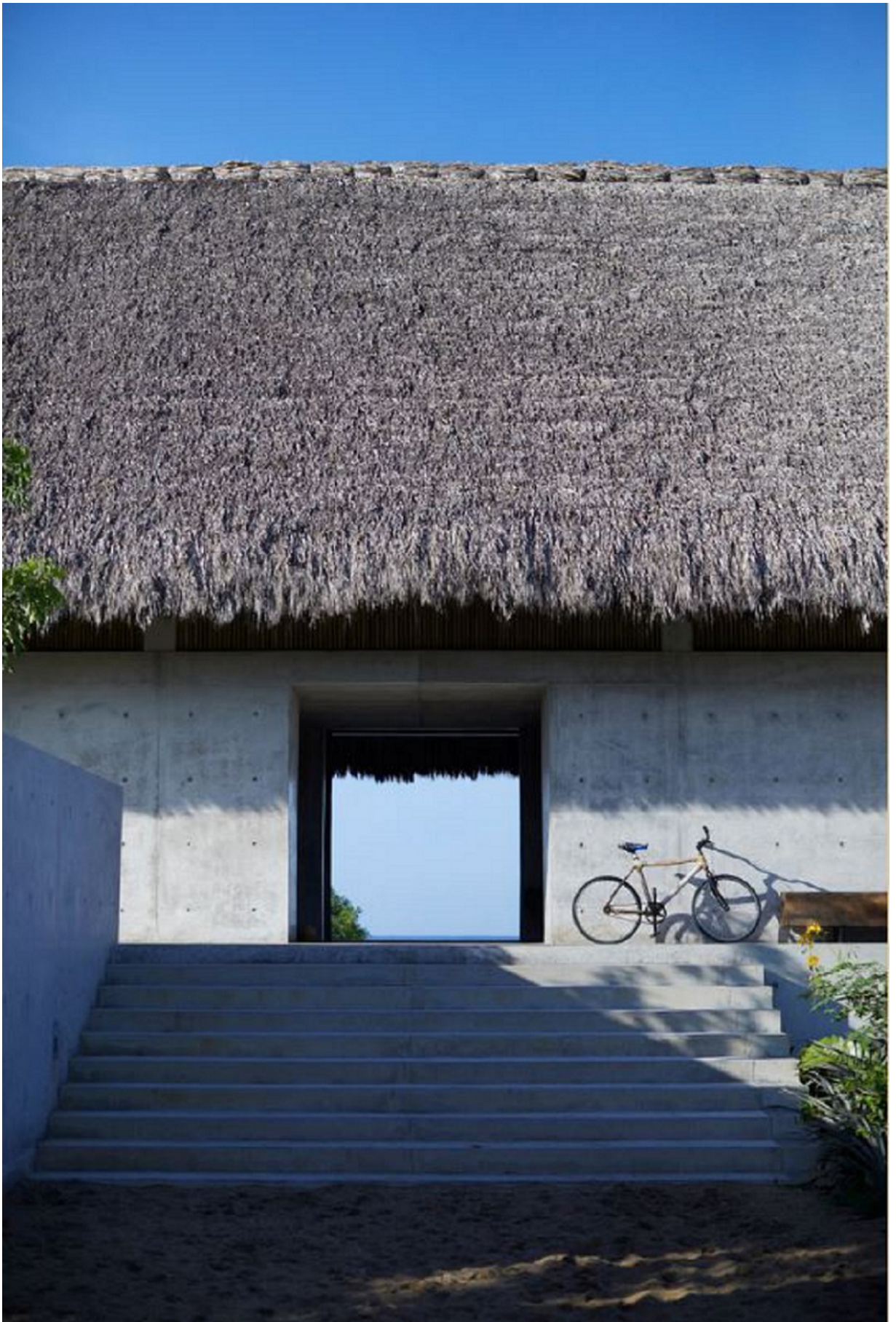
Fig. 3: Frontal view of the palapa thatched roof and access to the main building designed by Ando. Source: Sergio López, 2019. Available at: https://www.sergiolopez.mx/houses/casa-wabi . Accessed 02 May 2021.
