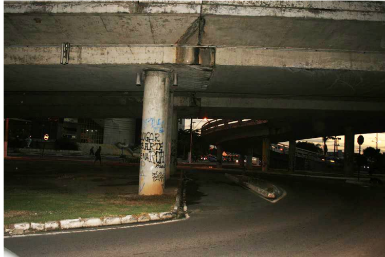
Fig. 2: Basement of D.I.A.'s Viaduct. Source: Author, 2017.
