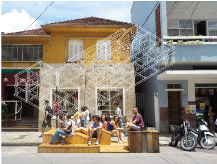
Fig. 8: Structural System. Source: Executive project produced by Gustavo Tristão, montage produced by Aleska Oliveira.
