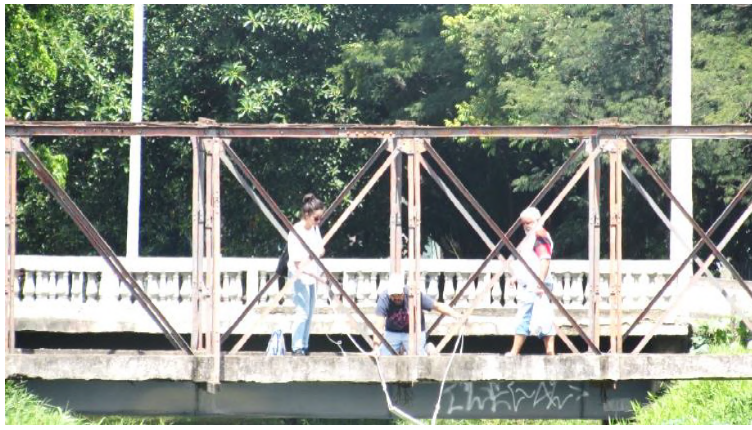
Fig. 8: Installation of the swing on the Biquinha Bridge. Source: Authors.
