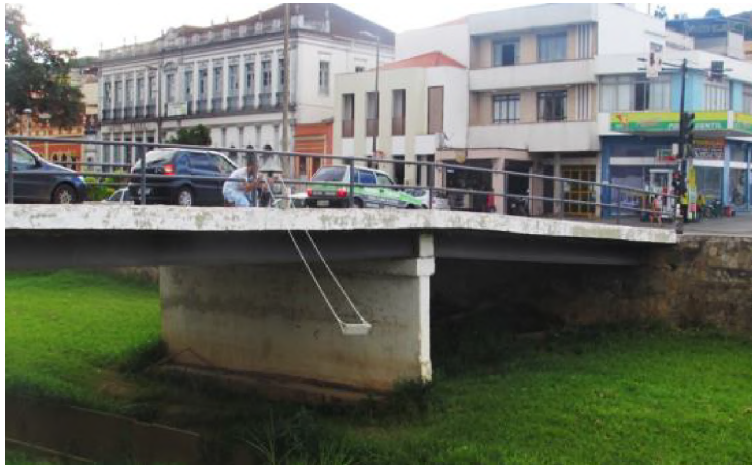
Fig. 10: Swing installed on the Estação Bridge. Source: Authors.
