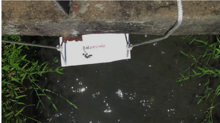
Fig. 9: Swing installed seen from above on the Cadeia Bridge. Source: Authors.
