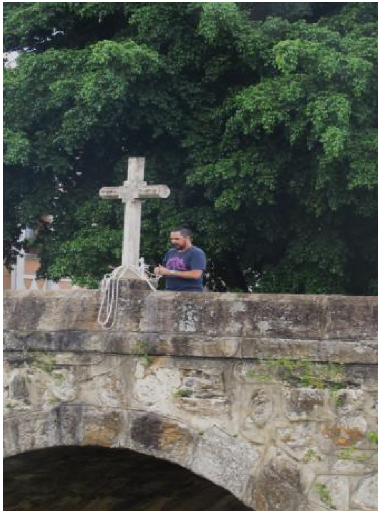
Fig. 11: Team member preparing to install the swing on the Rosario Bridge. Source: Authors.
