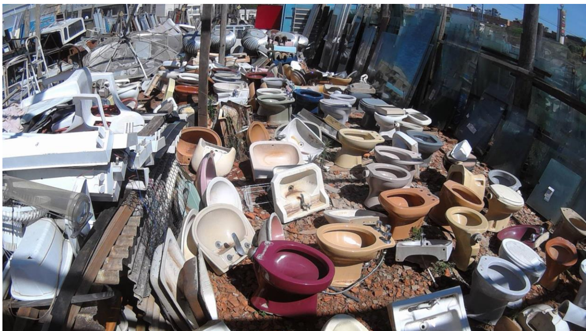
Fig. 1: Demolitions. Source: Nayara Benatti, Tássia Vasconcelos and Yasmin Bidim, 2016.
