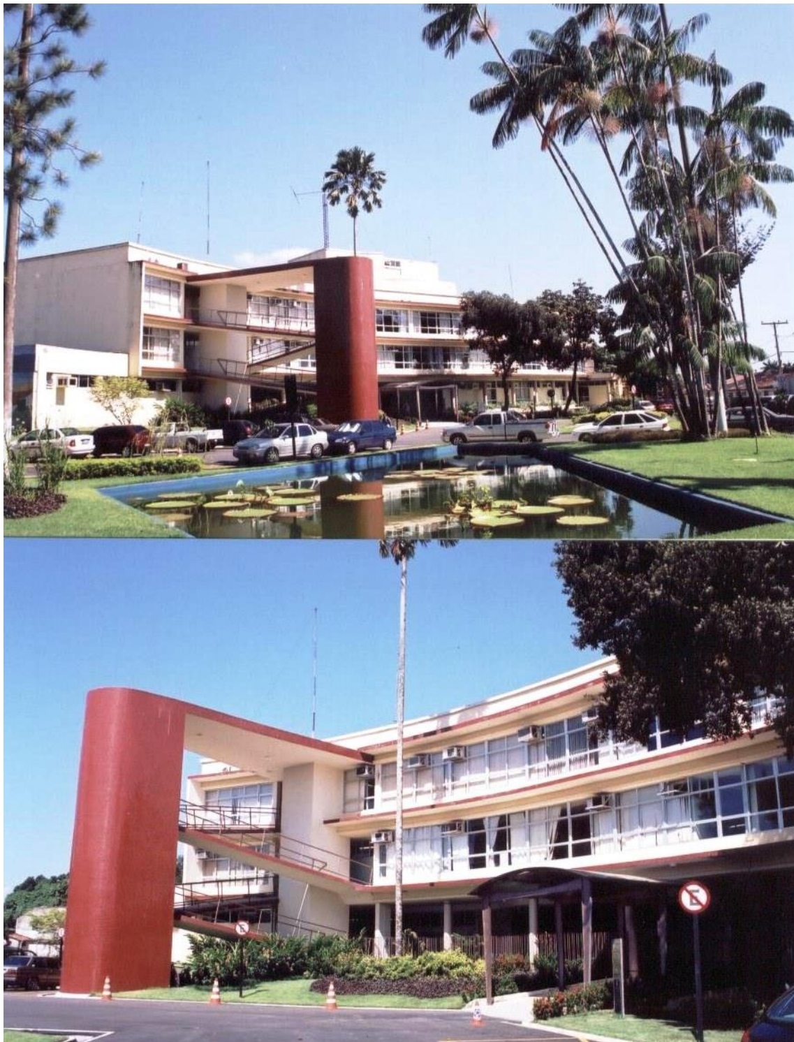
Fig. 14: Affonso Freire Building, 1949 (Headquarters of Secretaria de Estado de Transportes-Setran [State Department of Transportation] Pará, Belém, old Departamento de Estradas de Rodagem-DER [Department of Highways]). Camilo Porto de Oliveira. Source: Chaves (2006) – Setran, Pará, Belém.
