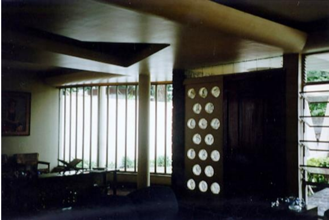
Fig. 6: Cobogó and brise soleil in the Bittencourt House (1950s). Camilo Porto de Oliveira. Source: Oliveira (2001).
