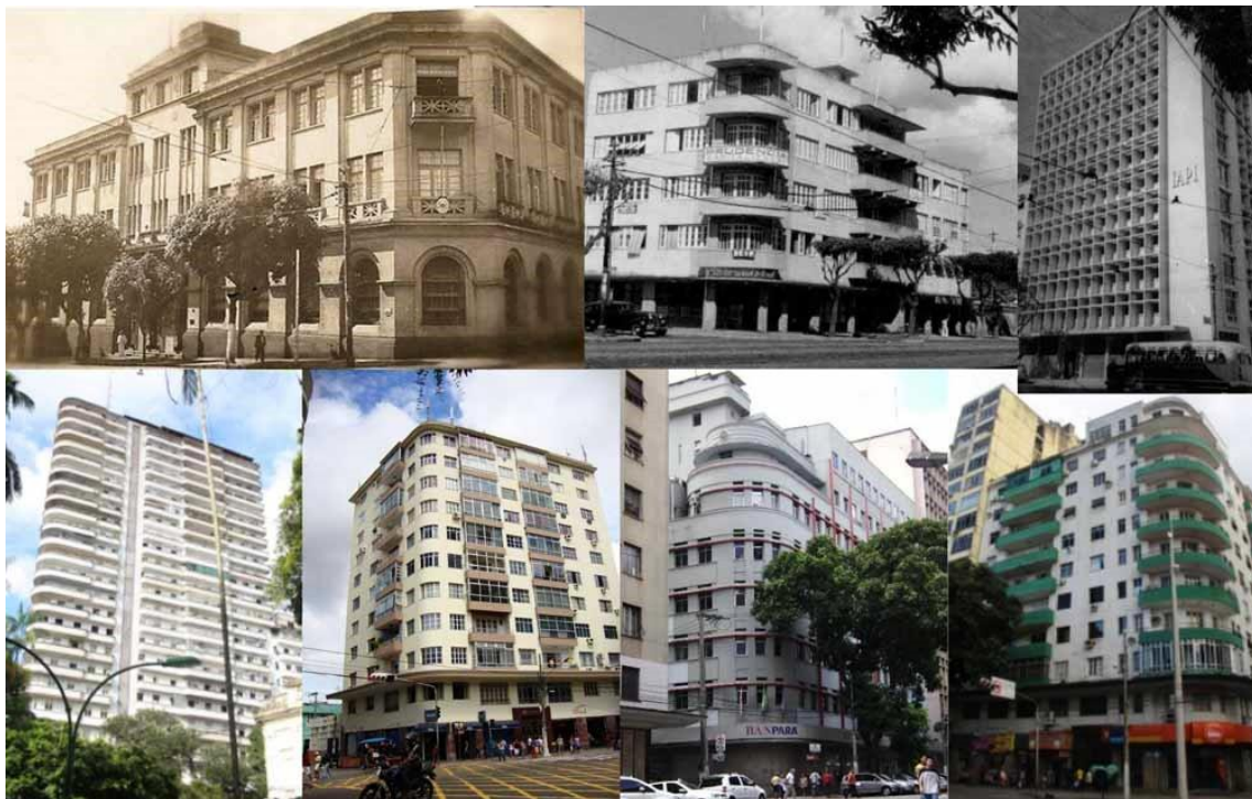
Fig. 2: Above, the buildings from left to right: Line Booth (1945); Bern (1940s); INSS (1958); Below, the buildings from left to right: Manoel Pinto da Silva (1960), Renaissance (1949), Dias Paes (1945), and Piedade (1950).
