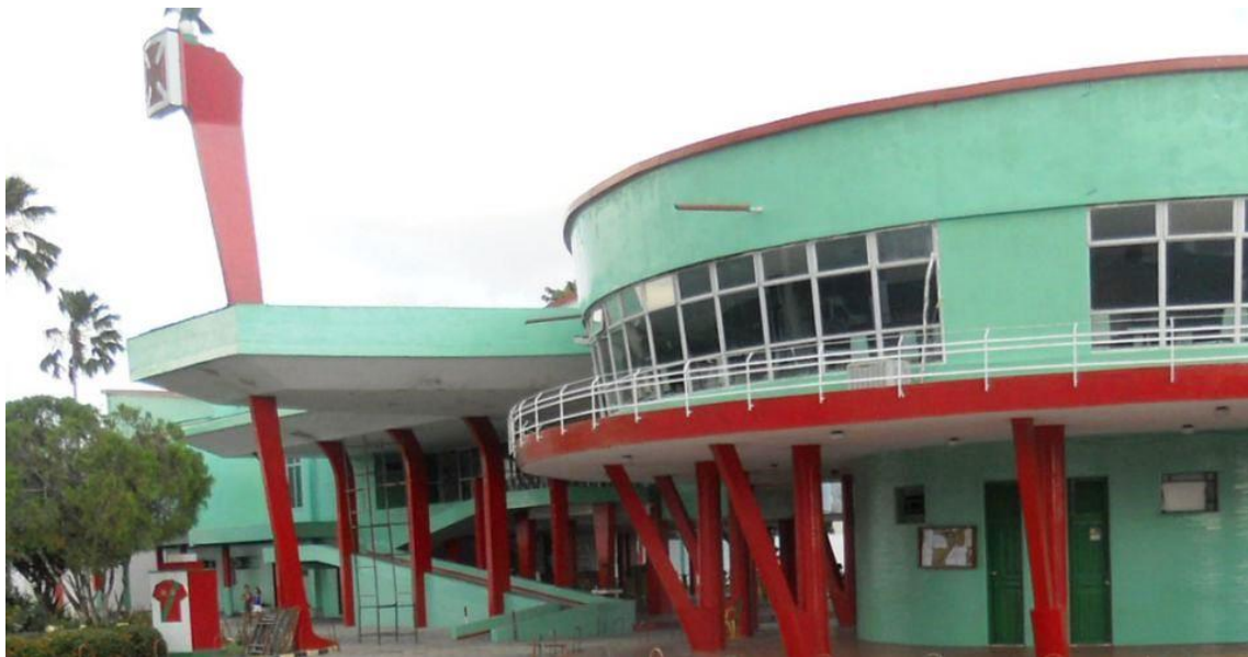
Fig. 17: Amorim Headquarters of Tuna Luso-Brazilian. Engineer Laurindo Amorim. Source: Hohlenwerger. Available at: < http://atat-pa.blogspot.com.br/2013/05/arquitetura-moderna-na-sede-campestre.html/ > [Accessed 21 May 2016].
