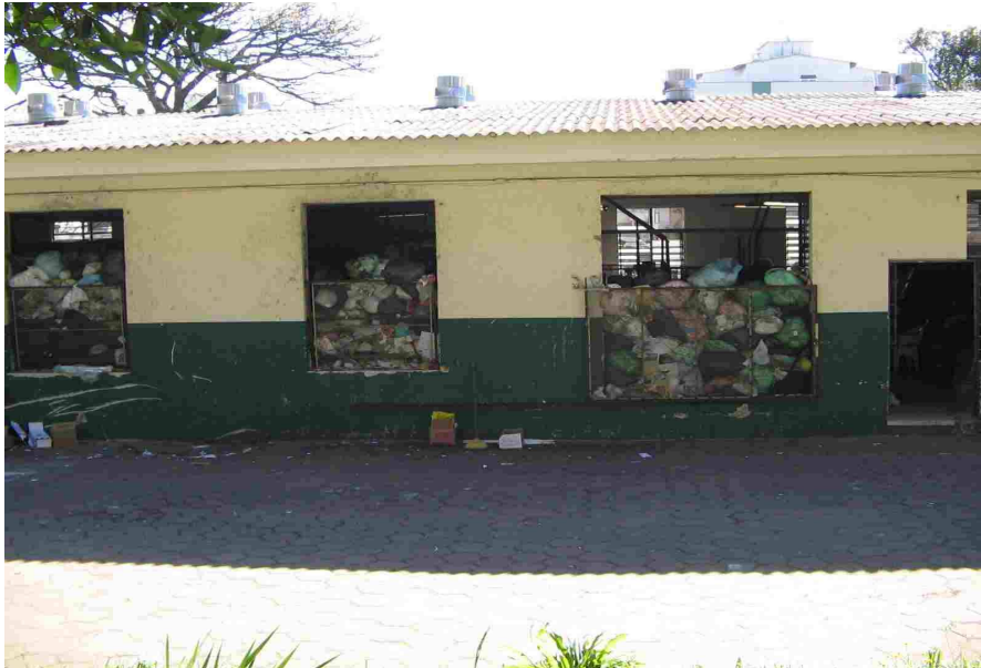
Figure 7: Outside view of the Waste recycling shed of the Hospital São Pedro . Photo by Bruno Cesar E. de Mello.
