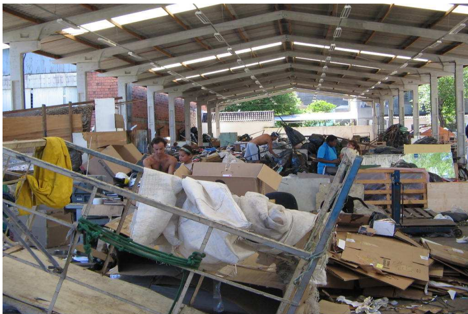
Figure 10: View of the AREVIPA Roofing. Photo by Bruno Cesar E. de Mello.
