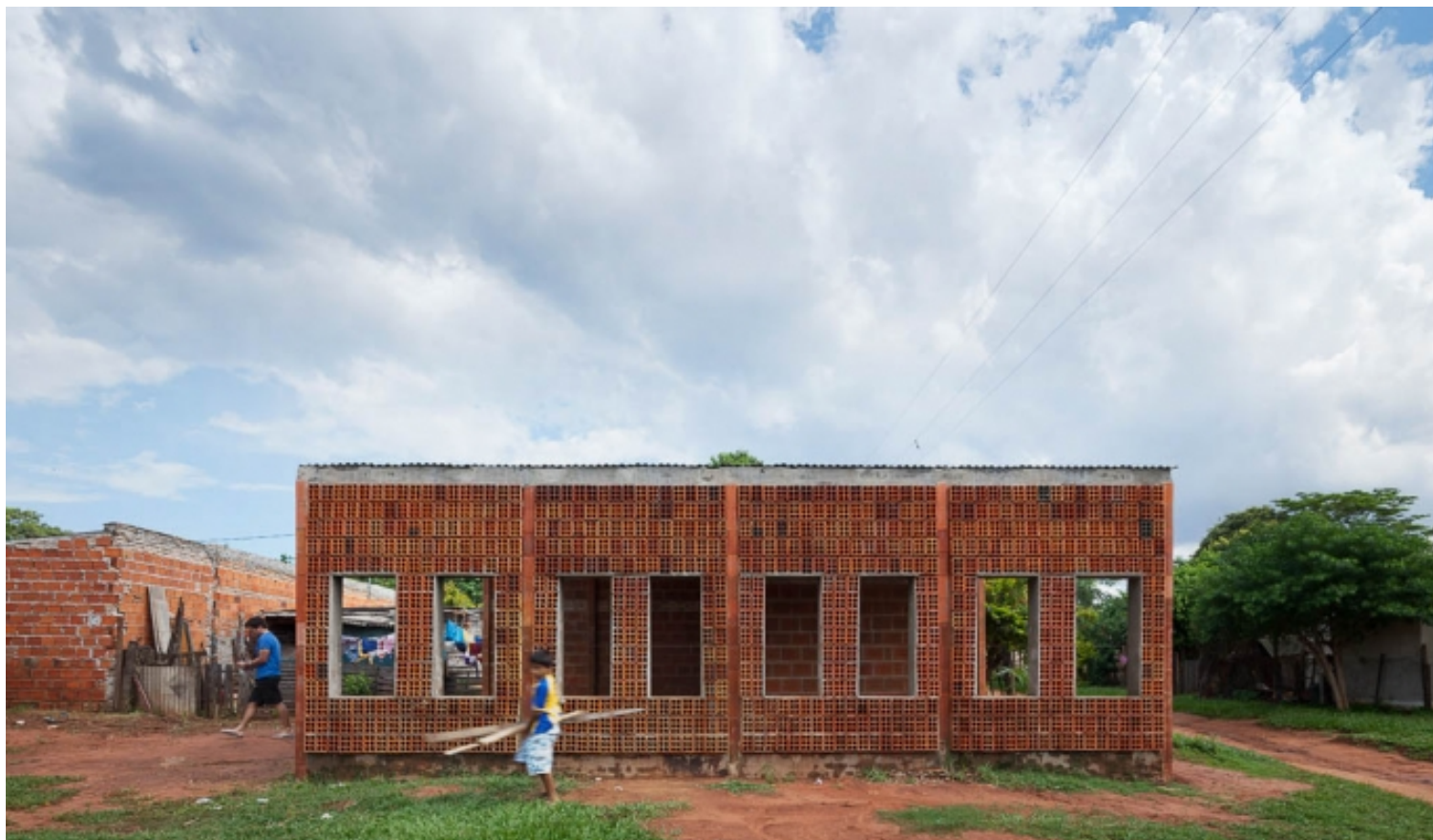
Fig. 2: Community Development Center, OCA + Bonini Arquitectos, Luque, Paraguay, 2014. Source: Federico Cairoli, 2015. Available at: http://www.federicocairoli.com/works/-centro-de-desarrollo-comunitario/ . Accessed 27 Oct 2022.
