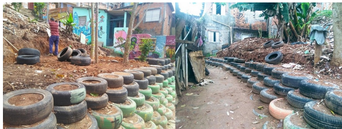
Fig. 15: Intervention in the lower plane of the terrain, performed with tires and debris from the site itself. Source: The authors, 2018.
