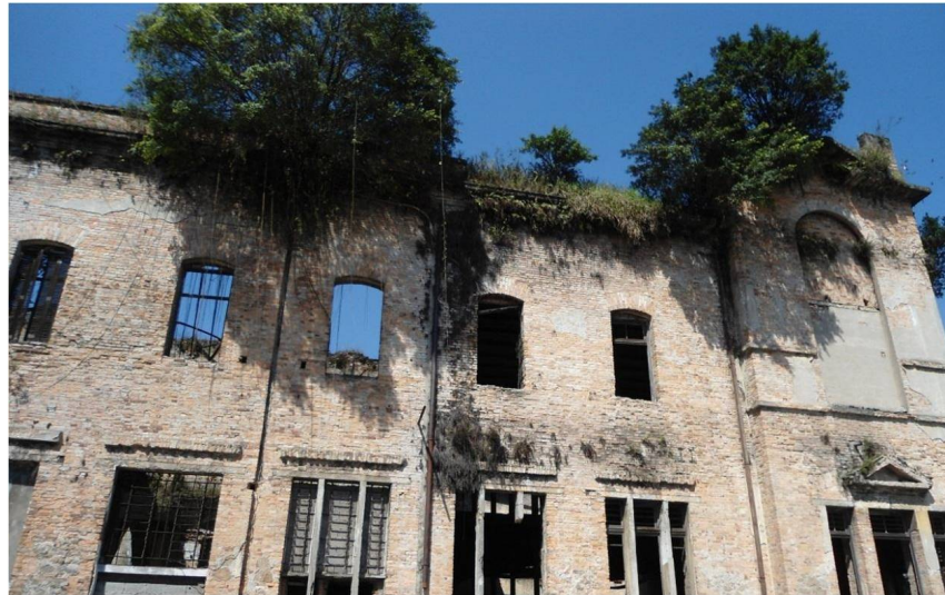
Fig. 5. Trees at the top of the north wing of the Hospedaria. Photo: Laís Hanson, 2012.
