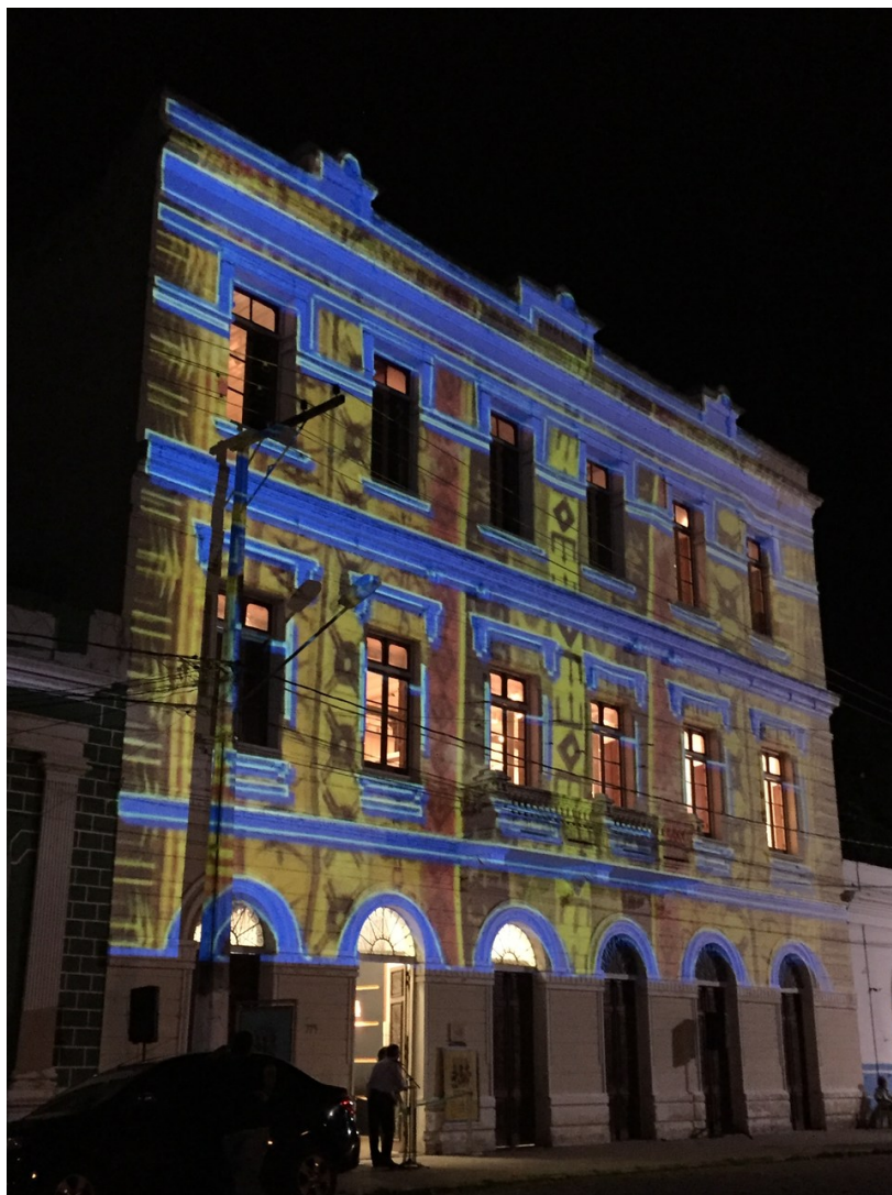
Fig. 8: Intervention in the MUHPAN building. Corumbá. Source: Sol Ztt, 2016.
