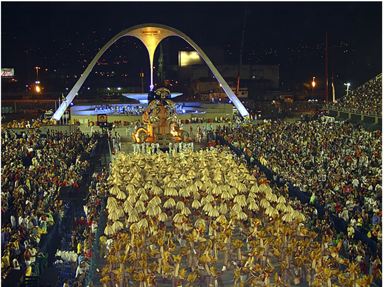
Fig. 3: It is possible to observe the angles of the arch forming a thong bikini. The Rio Samba Walkway. Source: Rio de Janeiro City Hall. Available at: http://www.rio.rj.gov.br/web/portaldoservidor/exibeconteudo?id=5048468 . Accessed 18 May 2021.
