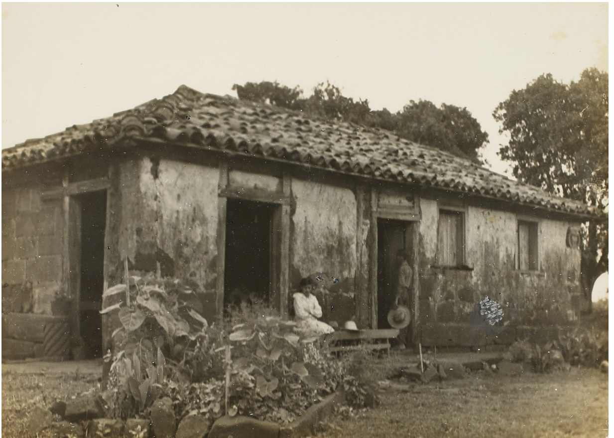
Fig. 5. House at Entre-Ijuís built with building material extracted from a Jesuit Reduction. [Demolished]. Source: IPHAN. Available at: www.ipatrimonio.org/entre-ijuis-casa-construida-com-material-missioneiro . Accessed 04 June 2021.
