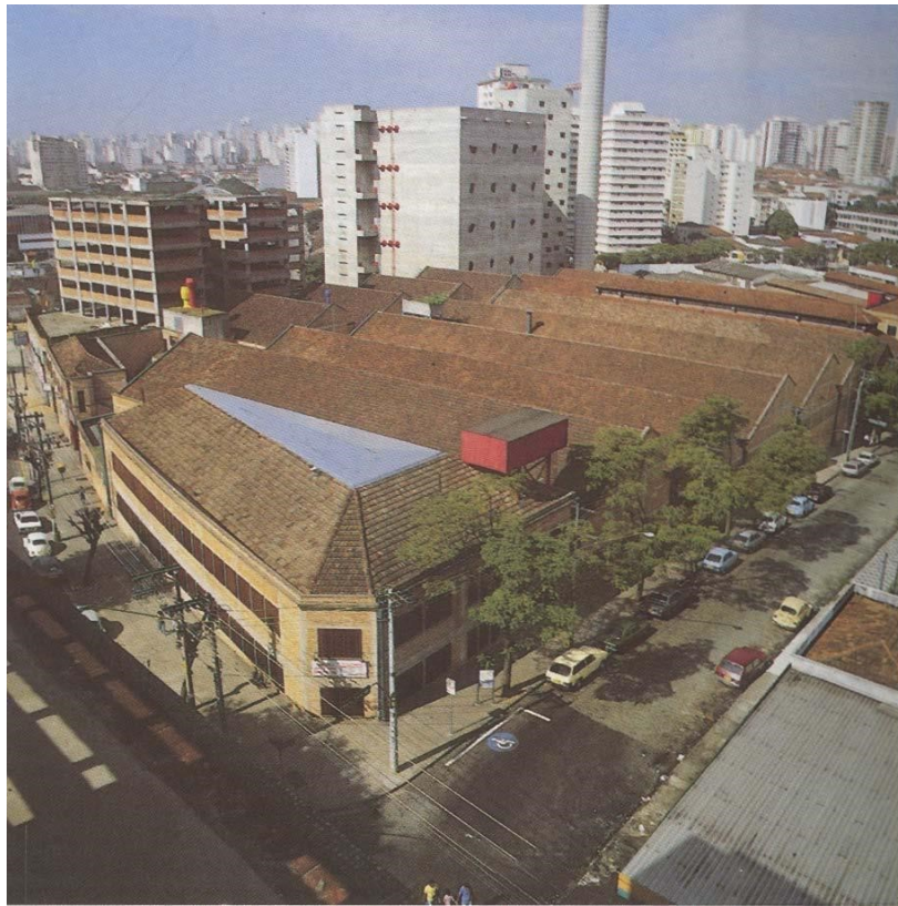
Fig. 4: View of the complex after Lina Bo Bardi's intervention. Source: Carvalho Ferraz (1994).
