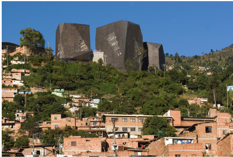
Fig. 6: Santo Domingo Library Park. Source: <plataformaarquitectura.cl/cl/02-6075/biblioteca-parque-espana-giancarlo-mazzanti> [Accessed 8 May 2017].
