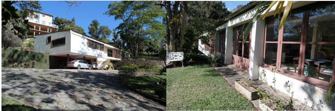
Fig. 8 e 9: Residence Guilherme Brandi, by Sergio Bernardes. Samambaia, Petrópolis. Building located by a student. Source: Silva, 2014.
