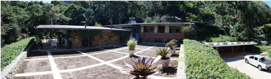
Fig. 5: Lota Macedo Soares House, by Sergio Bernardes. Located with the help of a student. Source: Silva, 2015.
