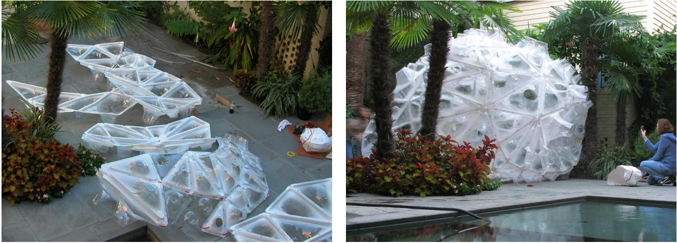
Figure 15. Groups of cells and exterior view after assembly.
