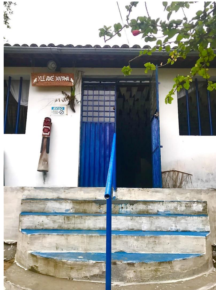
Fig.12: Entrance to the Shed. Source: Rodrigo Costa, 2021.
