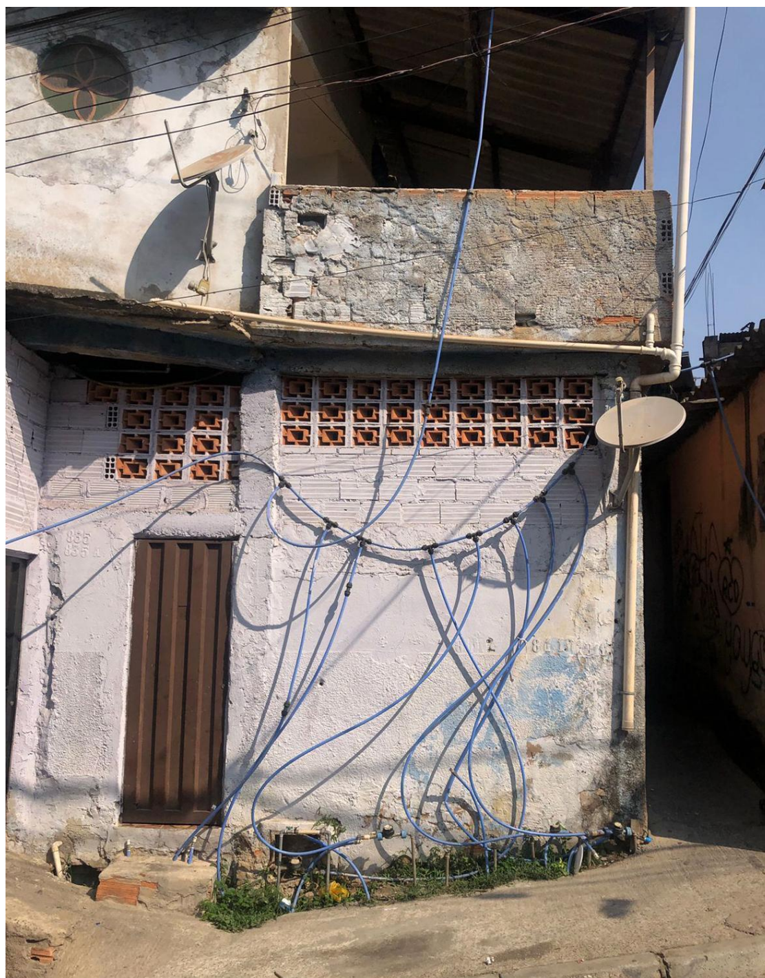
Fig. 3: Water connections exposed on a house facade at Pedreira Prado Lopes, in Belo Horizonte, a city located in the southeast of Brazil. Source: Author, 2022.
