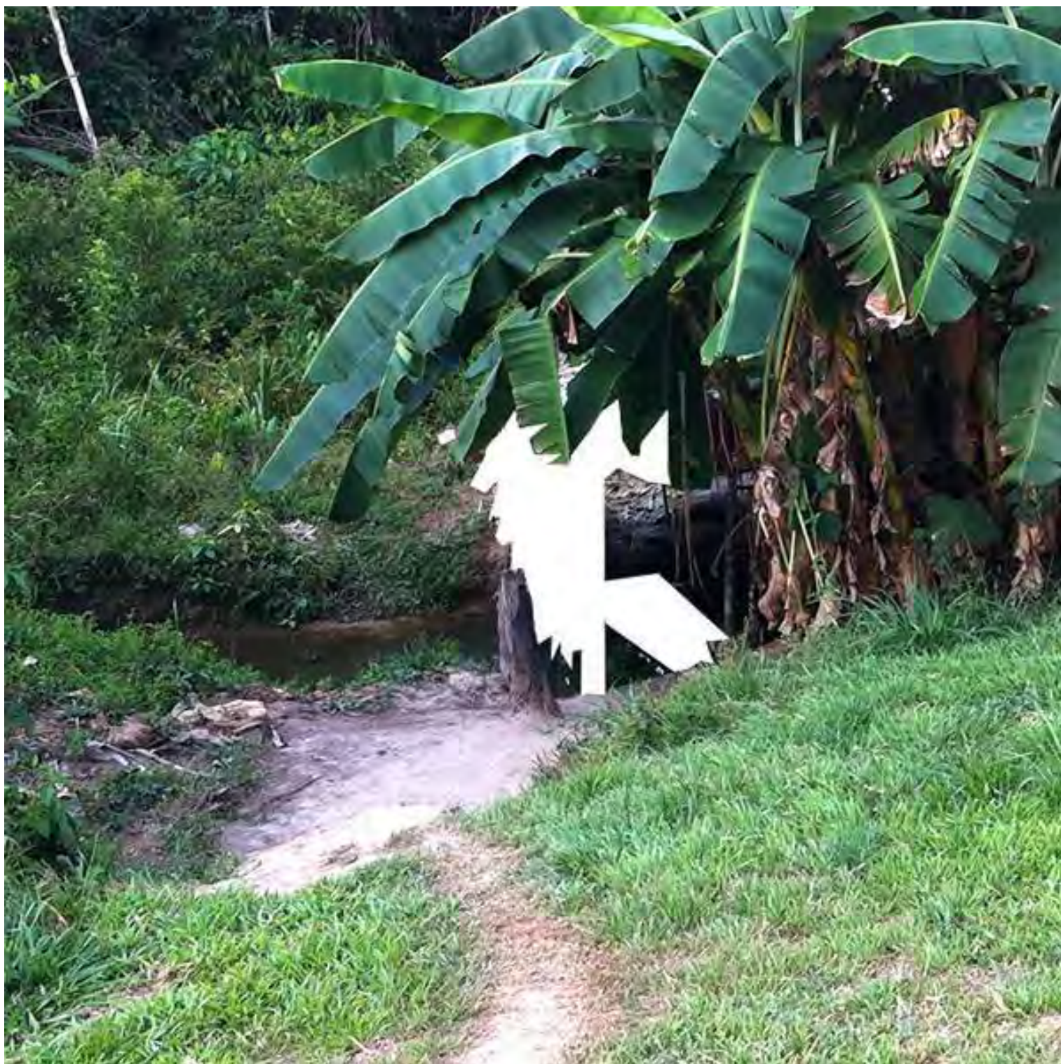
Fig. 13: Photographic record of the igarapé Mutum support structure. Source: Mendo, 2022 [photo, 2016].
