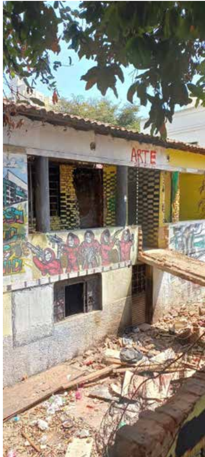
Fig. 1: House in Goiânia City (GO) used as mocó . Source: The authors, 2022.
