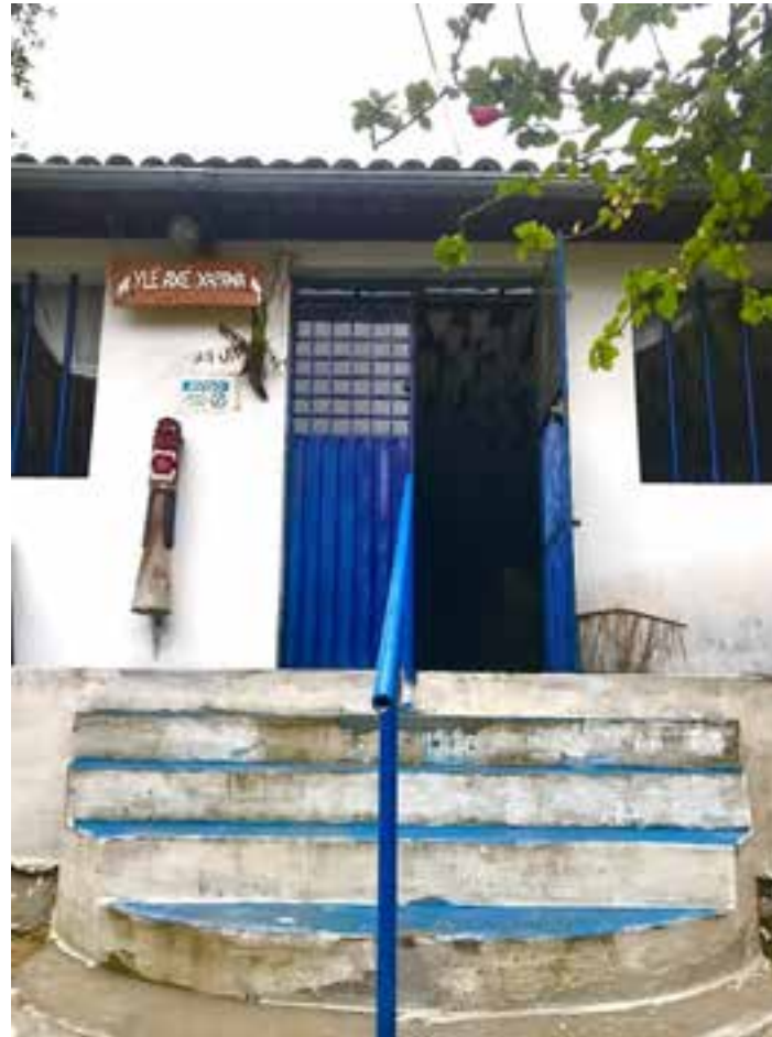
Fig.12: Entrance to the Shed. Source: Rodrigo Costa, 2021.
