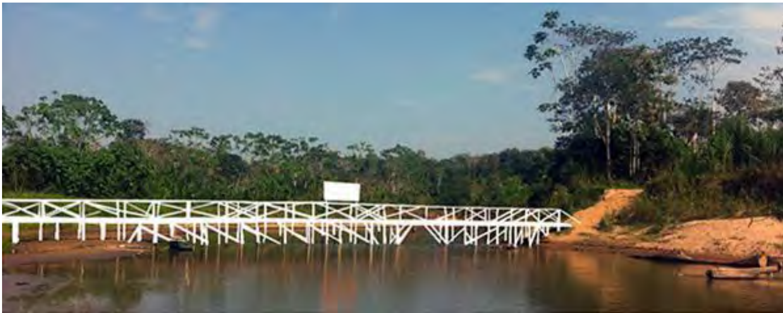
Fig. 12: Photographic record of the bridge built by the Yawanawá in Mutum village. Source: Mendo, 2022 [photo, 2016].
